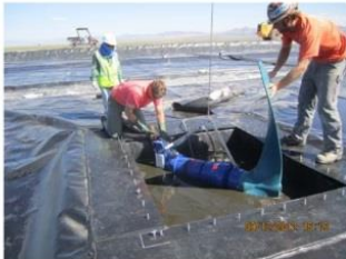
Installation of mixing equipment under gas cover.
