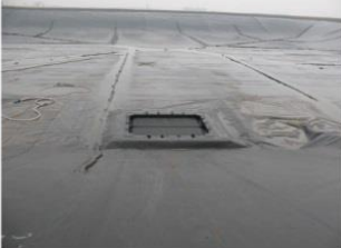
Completed hatch installation.
